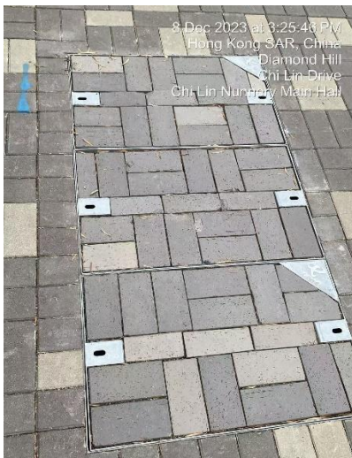
Joint Chamber (Recess Type)
