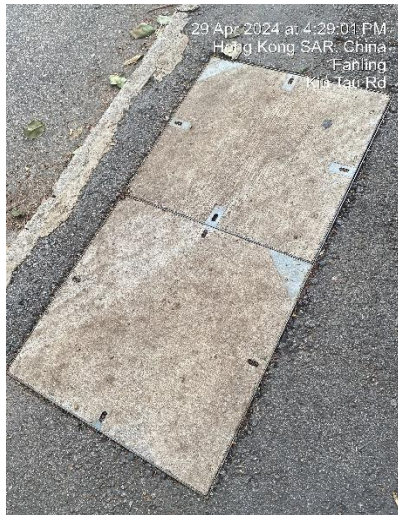
Joint Chamber (Concrete Type)
