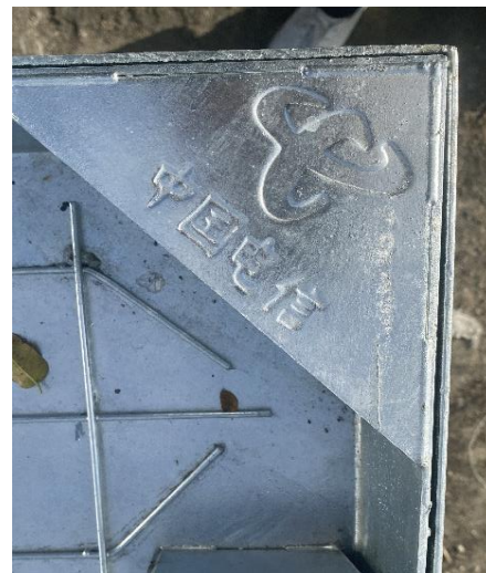
Joint Chamber (Recess Type)
